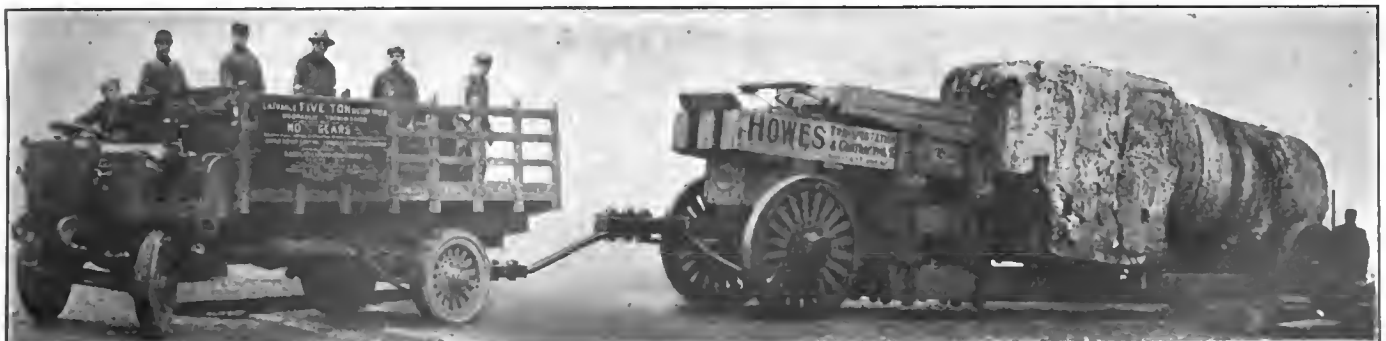
La France truck with hydraulic transmission hauling boiler weighing 23 tons. Truck weighs 12.5 tons
